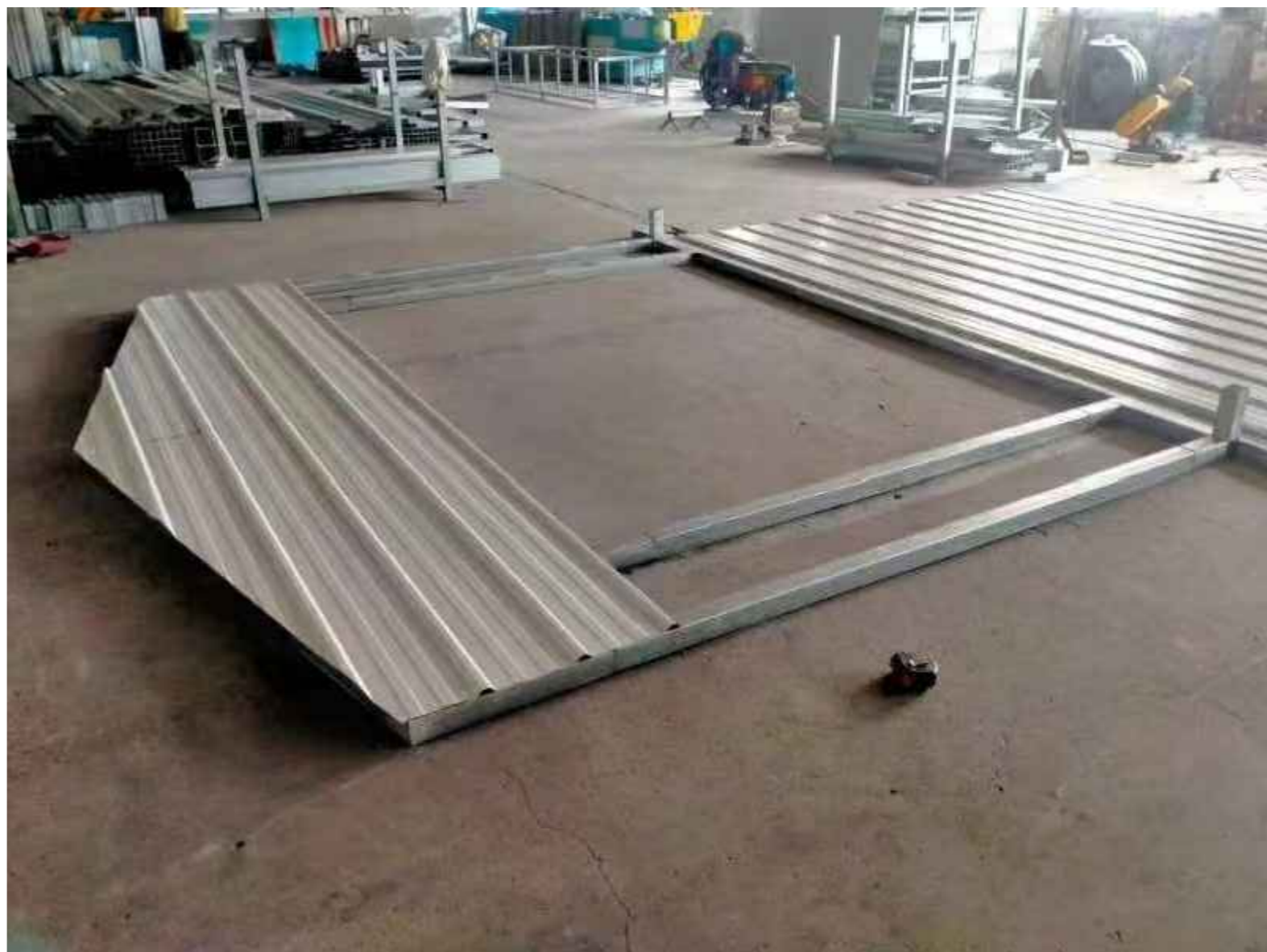
4: Install the roof panel from the roof center.
