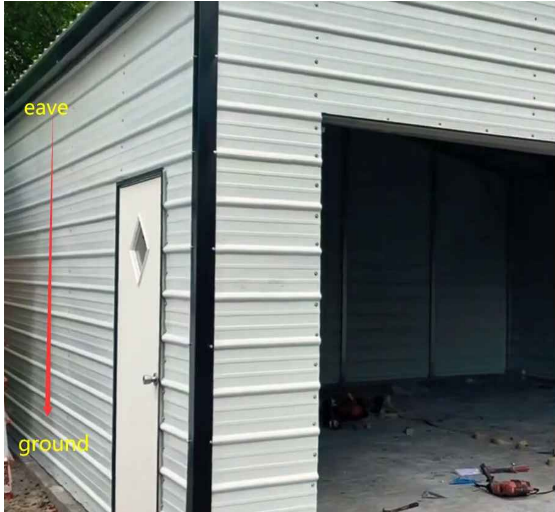
5: Install the side wall panel from the eave to the ground.
