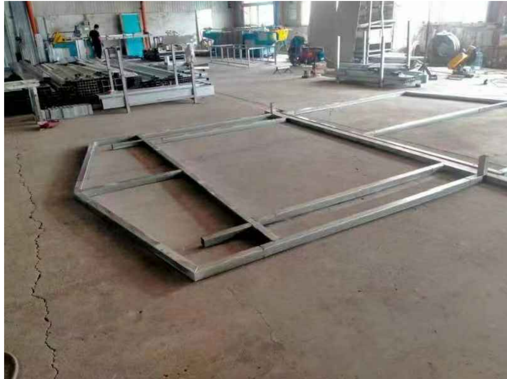
3: Install the whole garage steel frame structure.
